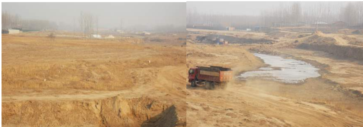
Juhe Restoration Project ; Photo taken by Hong Jianming on January 13, 2015
